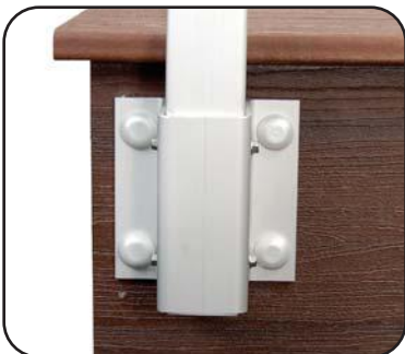
Finished fascia mount bracket with post installed.
