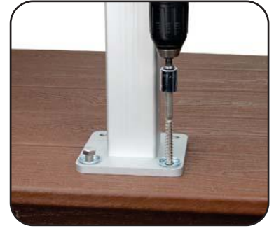
Step 3: Install cup washer under head of each fastener and drive fastener into blocking.
