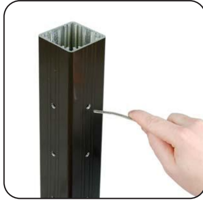
Step 2: Insert Cable Insert the cable into the hole and pass cable through the post. Make sure not to fray the end of the cable when passing through the post.
