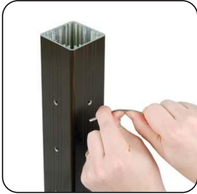
Step 1: Bend Cable Create a slight bend in the cable to allow for cable to more easily pass through the single corner post.
