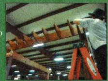
Install the Remaining long angle braces between the column and the bottom of the outside rafter on each corner, making sure that both angles set flat against the column and rafter. Fasten into place with the #7 x 2 -1/2" screws provided.
