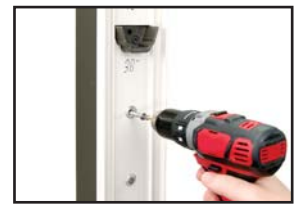
Fasten Threaded Connectors
