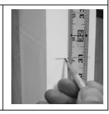
6. Align screw holes in the upper and lower saddle brackets (C&D) on the marked lines. Make sure the brackets are centered on the posts. Mark the screw hole locations with a pencil.
